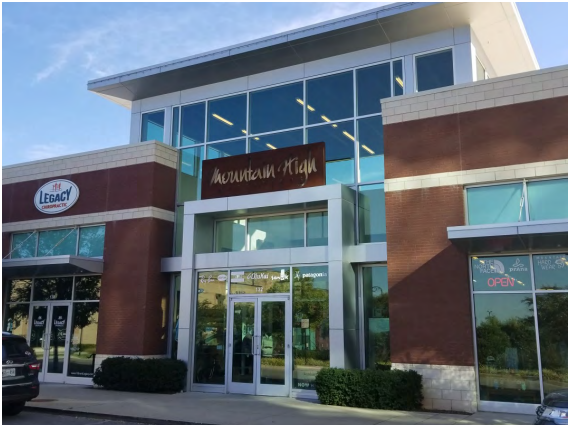
The building base is expressed with a different masonry material. The base at the storefront is expressed with an 8” raised bottom mullion.
