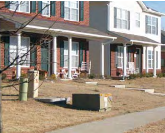
Utility boxes and pads should be consolidated at locations that can be screened (every 4-6 lots). This picture depicts inadequate screening
