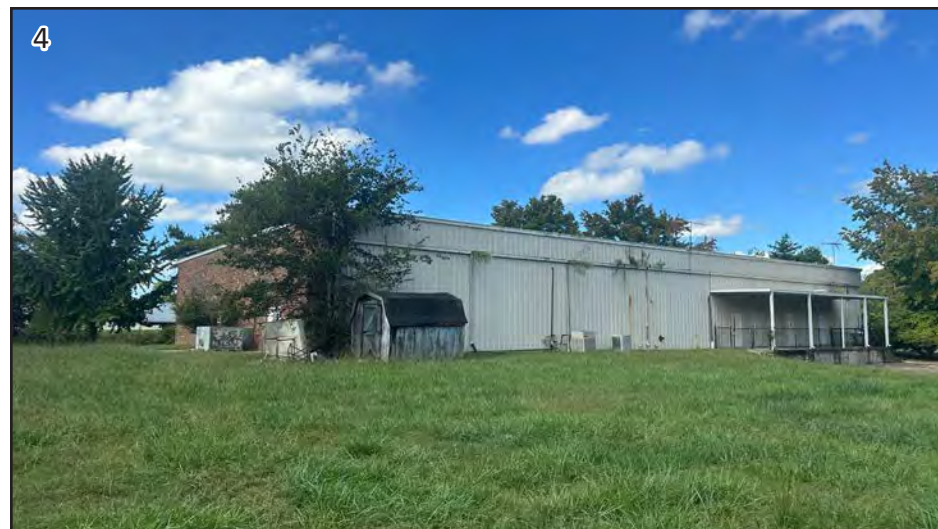
View of Existing Building On-Site Looking Northwest
